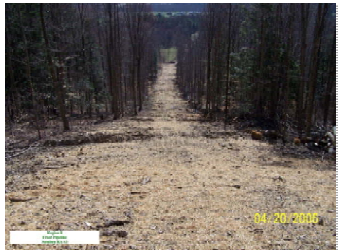
The Frost Pipeline on South Bradford State Forest in Steuben County exhibits the significant surface impact that must occur with pipeline development
