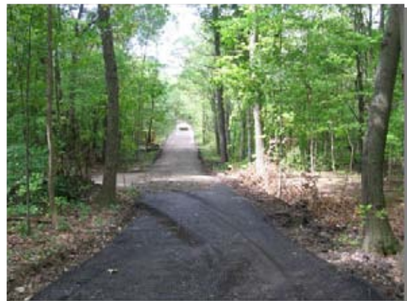
Road construction on Turkey Point State Forest in Ulster County
