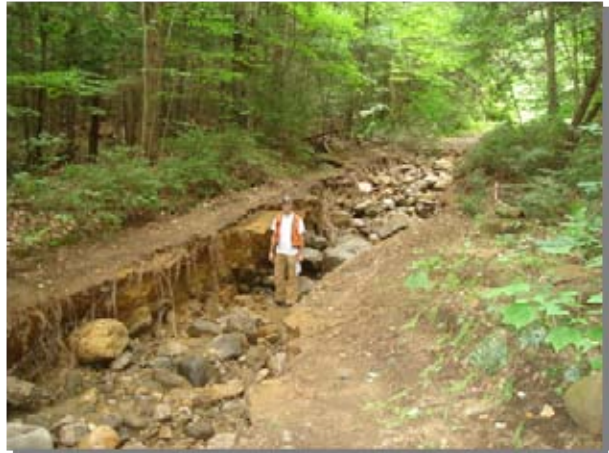
While this photo was not taken on State Forest lands, it illustrates that erosion problems can compound quickly when major storm events occur over exposed
