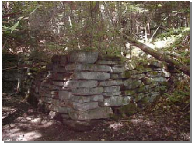
Sawmill foundation in Cattaraugus County
