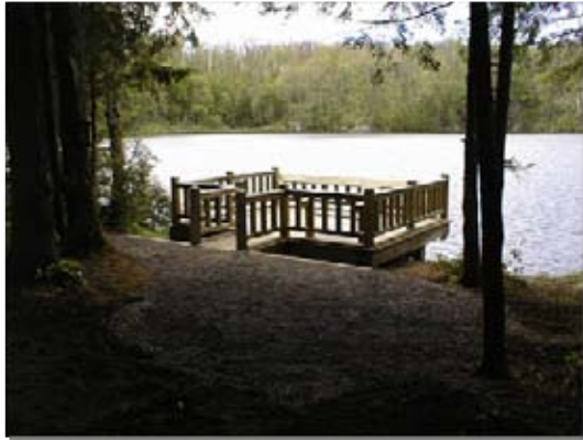
Accessible fishing pier and observation deck on Green Pond, Bonaparte's Cave State Forest in Lewis County, built using primarily natural materials
