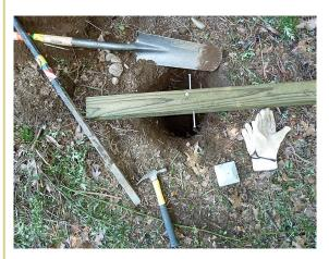
To prevent vandalism of the installed post, I drive four (4) 60d nails into the lower section of the post (see photo). I previously attached a cross member of 2 x 4 to the lower part of the post but have found that the nails seem to stand up to abuse better. Filling the hole with judiciously placed rocks and earth completes the job
